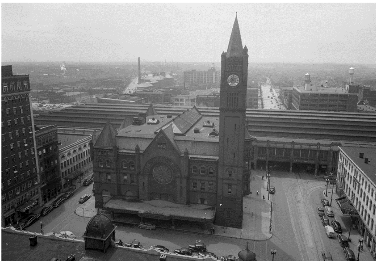
Indianapolis Union Station Headhouse and depot tracks Aug 1946 NYCSHS WR370424
