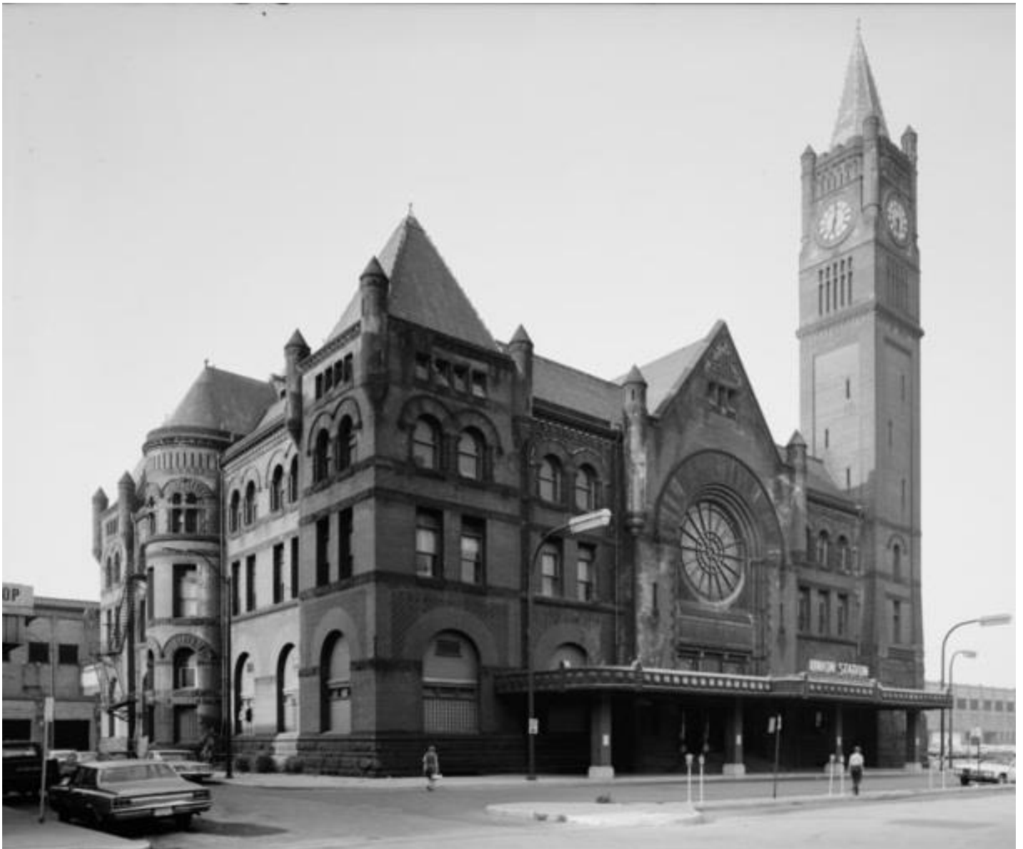
1880 Union Station headhouse c.1970 Library of Congress
