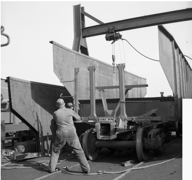
In the mid-1960s, Beech Grove crews converted 1948-1949 built offset-side, two-bay hoppers into Lot 942-H ribbed-sided hoppers. [NYCSHS NG525181 and NG525378]
