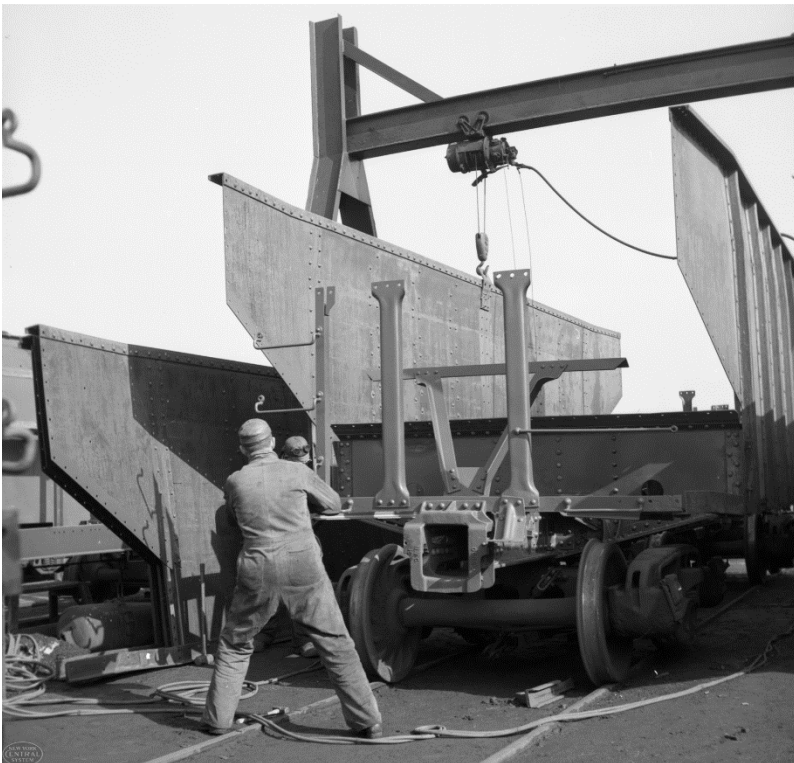
Crews were converting 1948-1949 offset-side, two-bay hoppers into lot 942-H ribbed-sided hoppers at Beech Grove in the mid-1960s. [NYCSHS NG525181 and NG525378]
