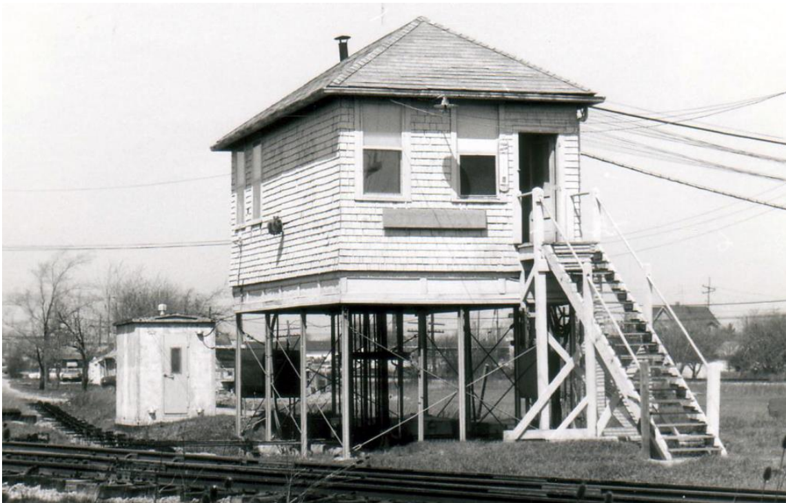
On the east side of town, where the main line split, was Gridley (GI) Tower. [Charles W. Bohi photo, NYCSHS Archives PB711151]
