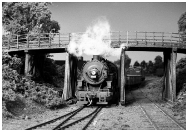
NYC no. 1415 works a factory lead in Adrian as she passes under the Center Street Bridge in Adrian. Photo by Doug Leffler
