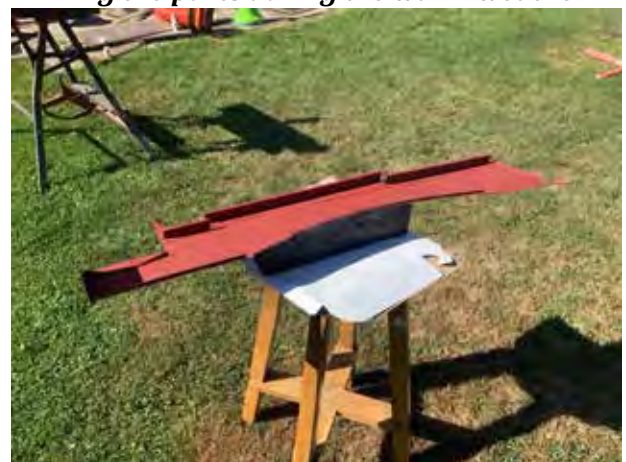
This time, both sides were primed and painted to prevent any rust forming.
