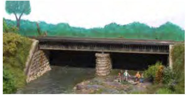
Chuck's completed model of the bridge after adjacent scenery was installed.
