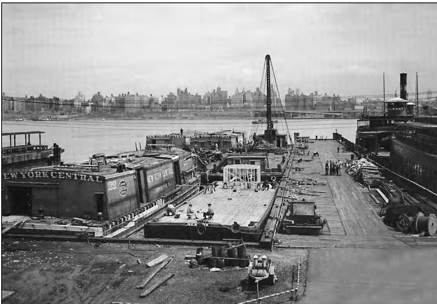
In this 1948 view looking out Pier 13 toward the river, we see two caulkers sitting on a wooden scow, while a carpenter labors on the cabin framework. At left, two more carpenters are doing roof repairs on the refrigerator barge Vernon . A carfloat is tied up on the north side of the pier, and two ferryboats, Albany and probably Stony Point , languish on the right side. An impromptu conference appears to be taking place halfway out the pier. Photo by Ed Nowak.
