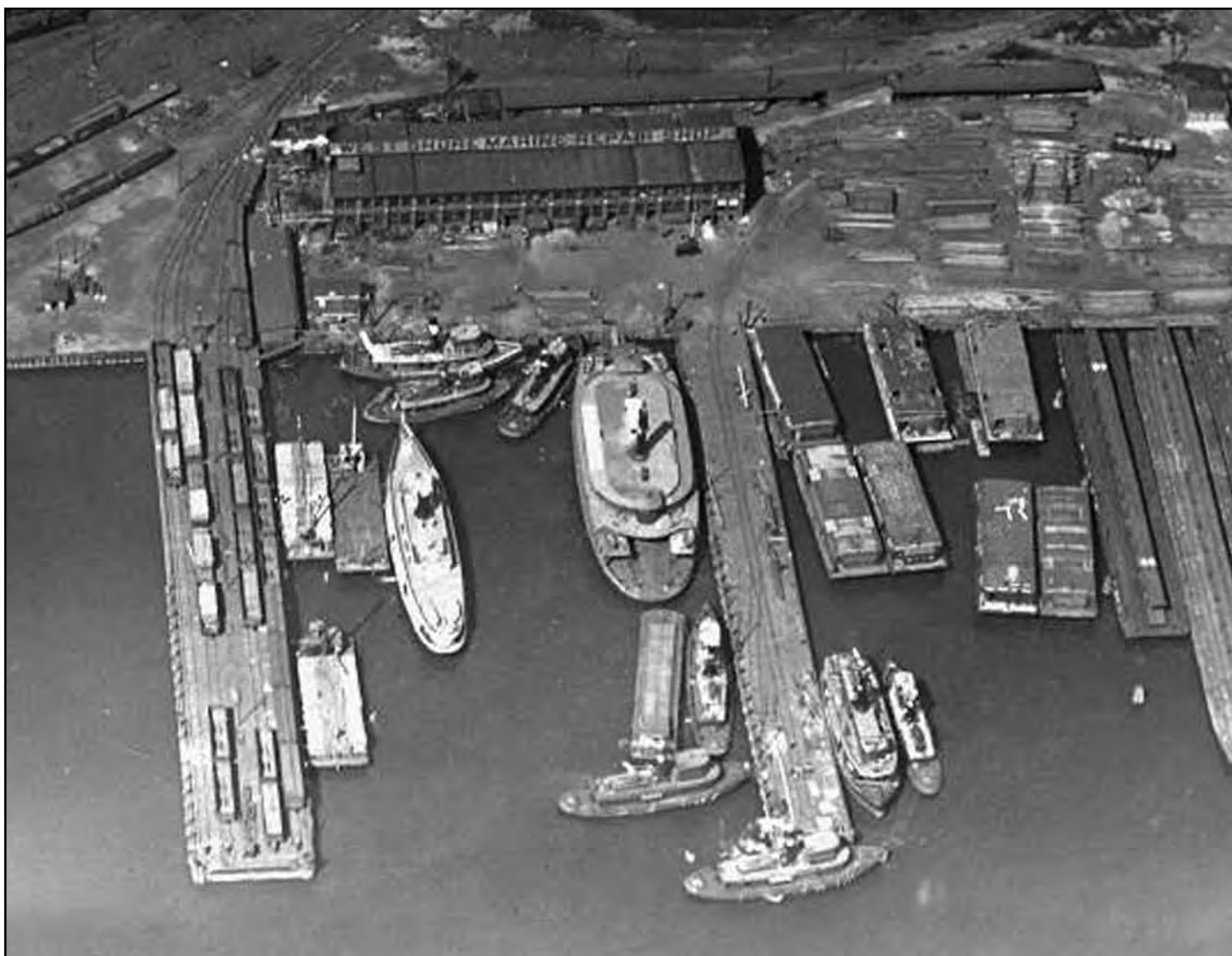
The Marine Repair Shop at West New York, New Jersey appears in this detail from an aerial photograph taken on September 18, 1922. Several craft are tied up between Piers 12 and 13, the largest being one of New York Central's eight ferryboats. NYCSHS Collection.
